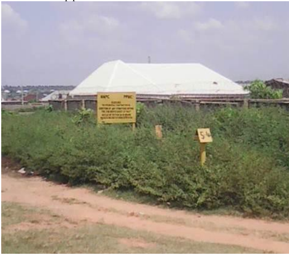
Plate 1: Encroachment by Residential Buildings on PROW along kilometer 2 site light town, Lagos pipeline right of way
